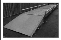
A low profile weighbridge that is versatile and easy to install, the structure is almost identical as the former. But because it is elevated and installed on the ground level, maintenance works are far easier. It also requires minimal and simple civil works.
