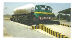
A low profile weighbridge that is versatile and easy to install, the structure is almost identical as the former. But because it is elevated and installed on the ground level, maintenance works are far easier. However, the land required for this is more as the approach ramps on both ends are a must.
